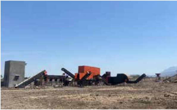
Figure 25: Auto-segregation facility at Ivnagar
